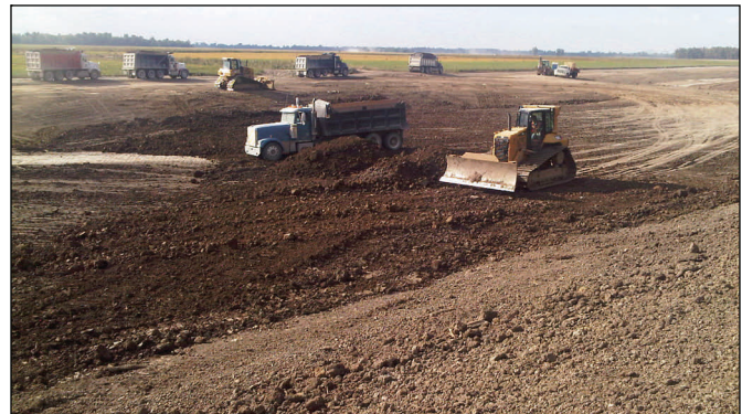
Clay embankment is placed in the final scour hole at the upper crevasse Monday to prevent seepage.
