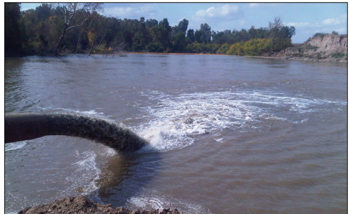
Sand dredged from the Mississippi River is pumped into the scour hole at the center crevasse Monday.
