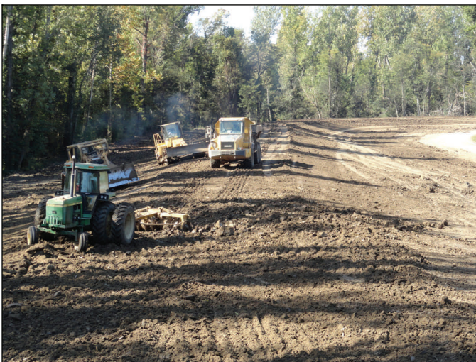
Constructing the final 1,200 feet of levee at the lower crevasse Monday. There is continuous levee now the entire length of the crevasse.
